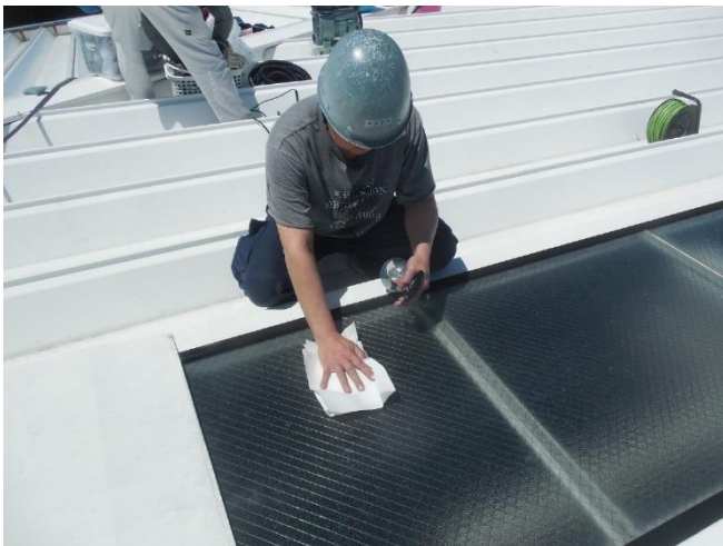
③ Cleaning (using silicon-off)
