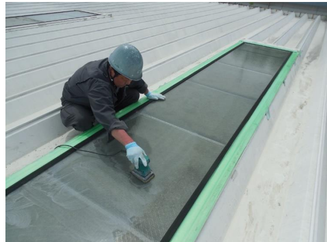
④ Cleaning (Using glass compound)
