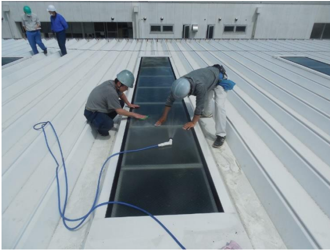
① Cleaning (Remove muds & dirt)
