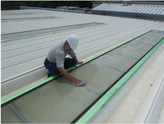
⑤ Cleaning (Remove Glass compound )
